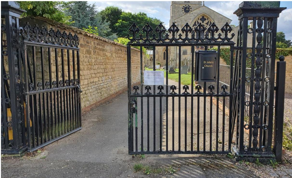
There is no requirement for any welding or drilling of the gate metalwork. The post box attaches via a simple clamp plate. The existing fabric of the gate will not be affected in anyway.
